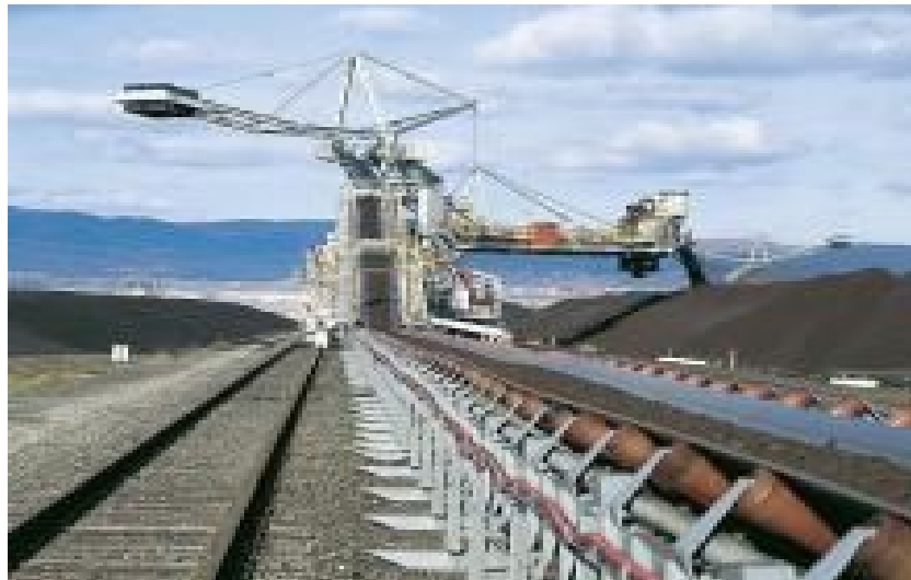
Stacker reclaimer in stacking
